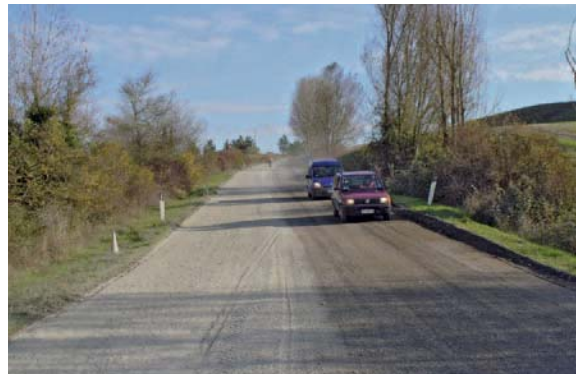
Recycled lane can be used after compaction.
